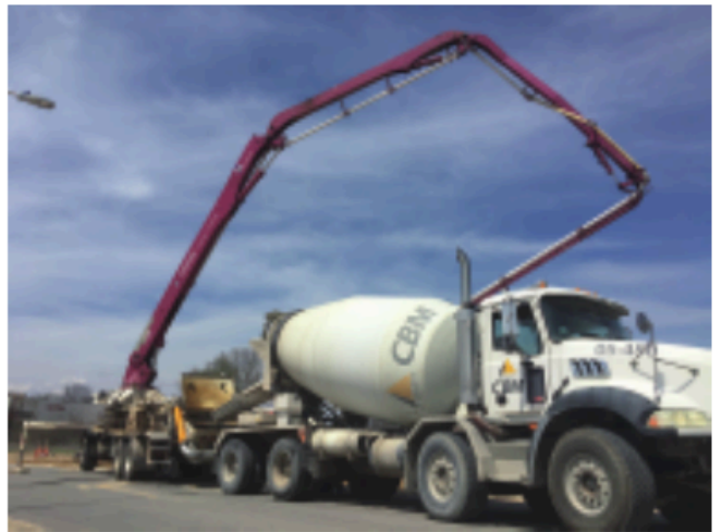
Concrete Pump Truck
