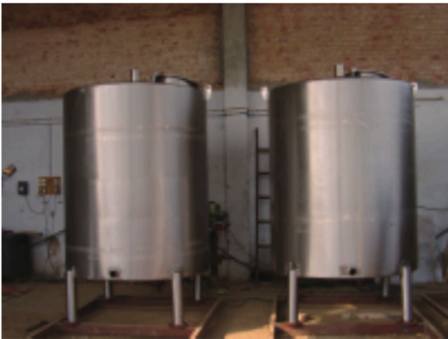
Pulp & Cement Storage
