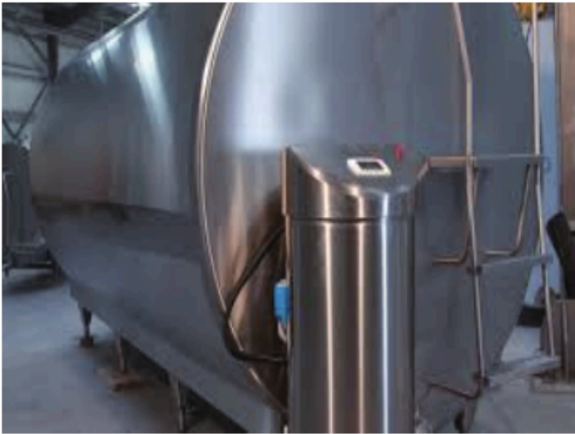
Milk Oil Storage Tank Monitoring
